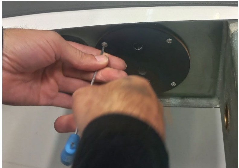
Figure 2 - Opening inspection hole
